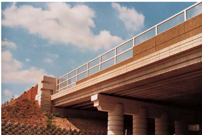
Sound barrier (Amien, France) Year: 1996 Material: Makrolon® UV, 8 mm
