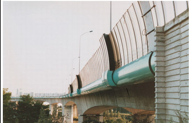
Sound barrier Bünde (Germany) Year: 1992 Material: Makrolon® UV, 12 mm
