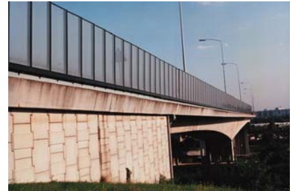
Sound barrier Pont de Genevilliers (France) Year: 1995 Material: Makrolon® UV, 10 mm
