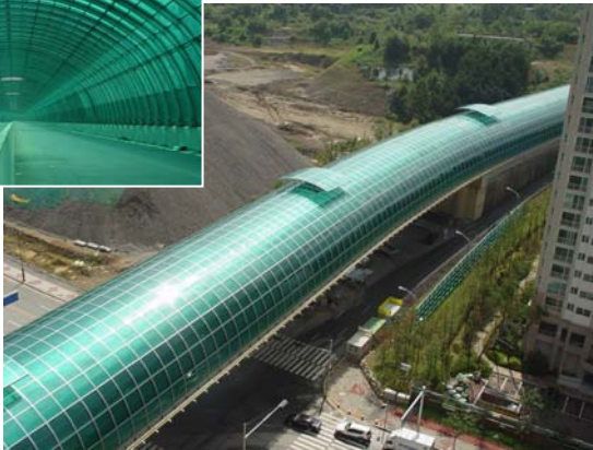
Sound barrier Seoul (Korea) Year: 2004 Material: Makrolon® UV, 12 mm
