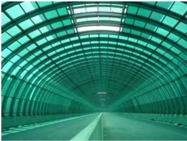
Sound barrier Seoul (Korea) Year: 2004 Material: Makrolon® UV, 12 mm
